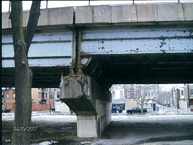
US 1 Wayne Ave. Viaduct, Phila.
