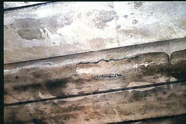
Holmes Ave. Bridge Over Route 1, Phila.
