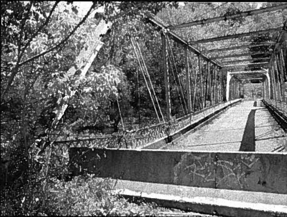
Gravel Run Rd. Bridge Crawford County
