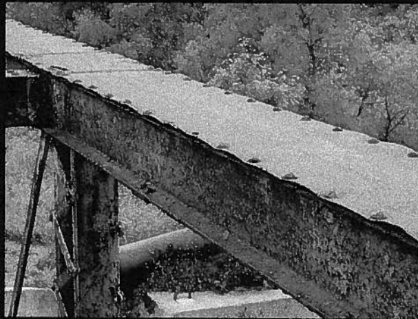
Mercer Pike Bridge Crawford County
