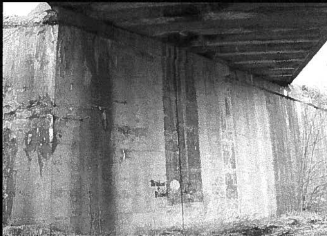
US 119 Home RR Bridge Indiana County
