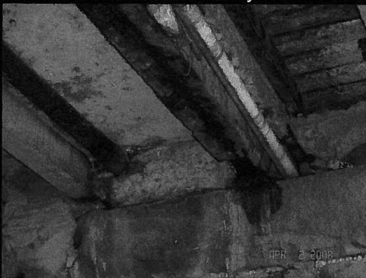
PA 36 Sawmill Run Bridge Jefferson County
