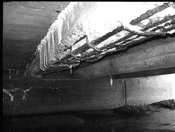
US 219 Crenshaw Bridge #1 Jefferson County
