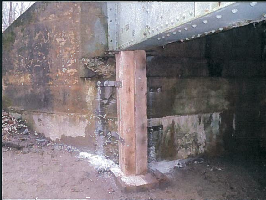
Fishing Creek Road Bridge, District 8
