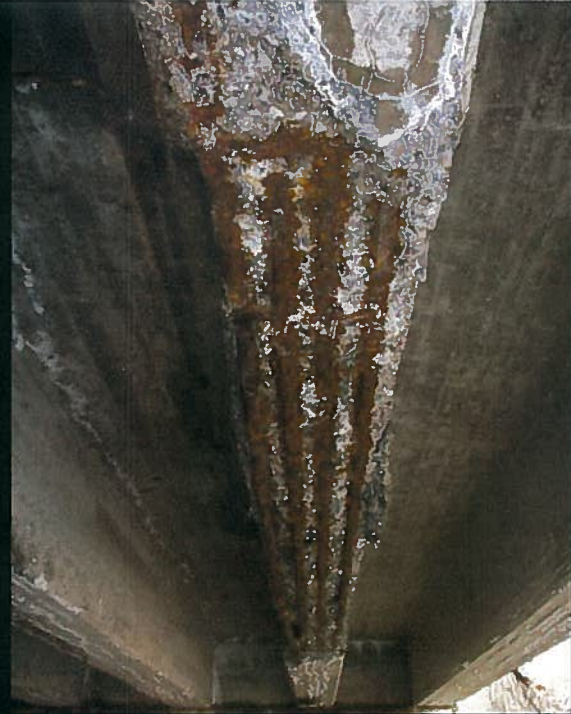
Route 654 over Mosquito Creek, District 3
