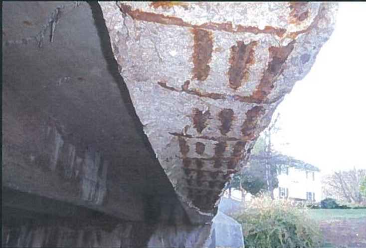
Route 2004, Fair Grounds Bridge
