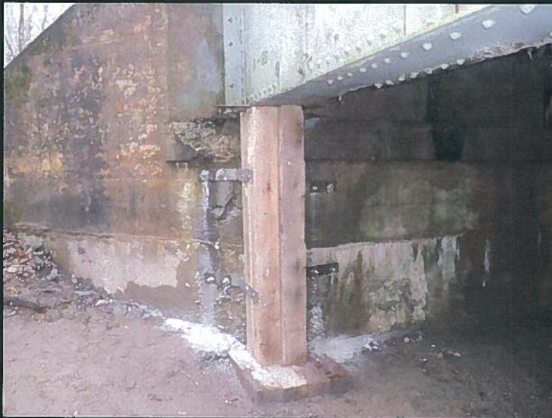
Fishing Creek Road Bridge
