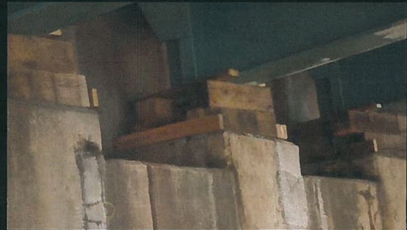
Route 322 Ramp Bridge in Eisenhower Interchange
