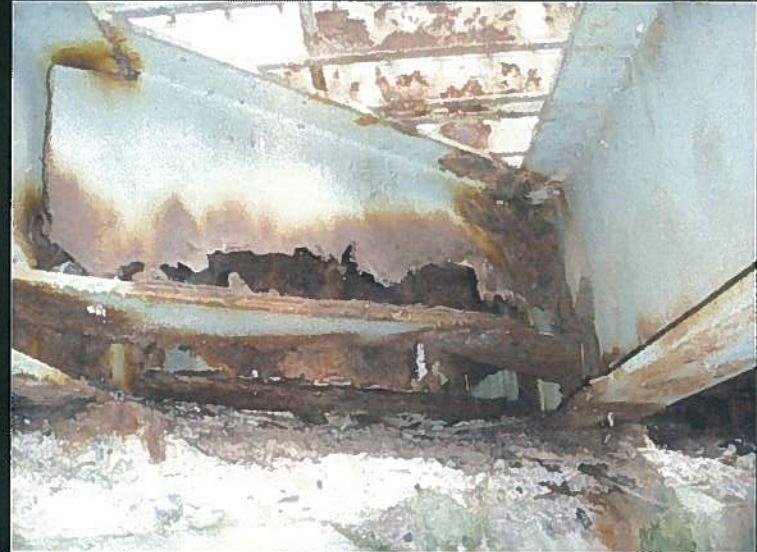
Clearview Drive Bridge
