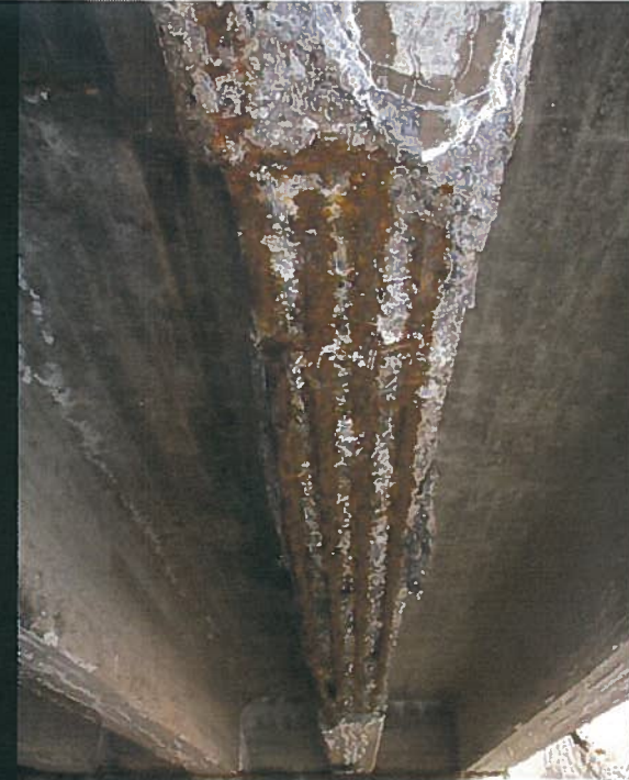
Route 654 over Mosquito Creek, District 3
