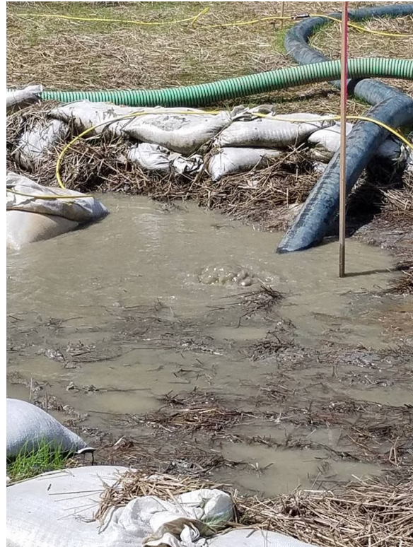
Frackout at Tunbridge Apartments, Middletown Township, Delaware County
