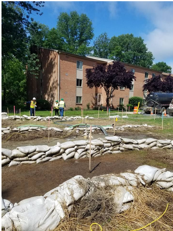
Frackout at Tunbridge Apartments, Middletown Township, Delaware County
